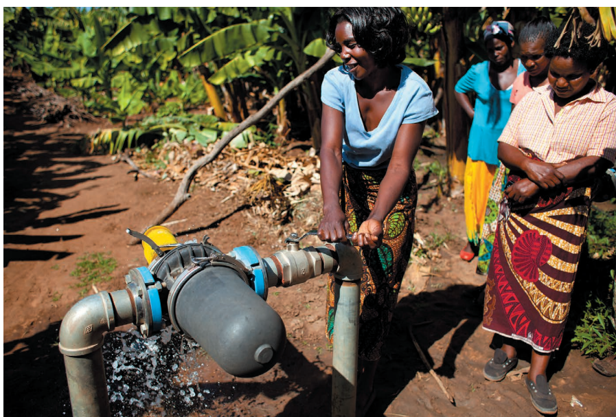
A hydro-powered irrigation pump in use at the Kabwadu Women's Banana Farm in Zambia.
